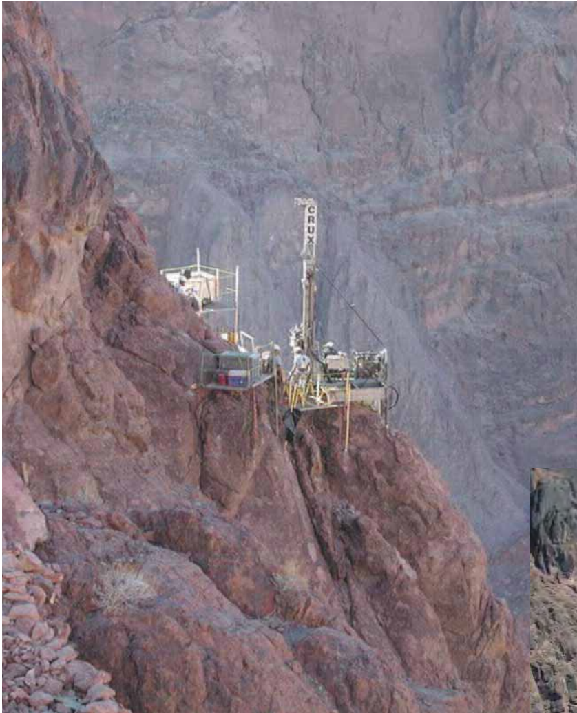
Drill rig is positioned on platforms for R13.
