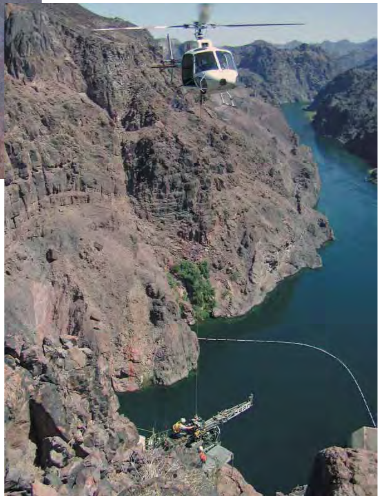
Another view of the helicopter and ground crew placing drill rig components at the Nevada Skewback Location.
