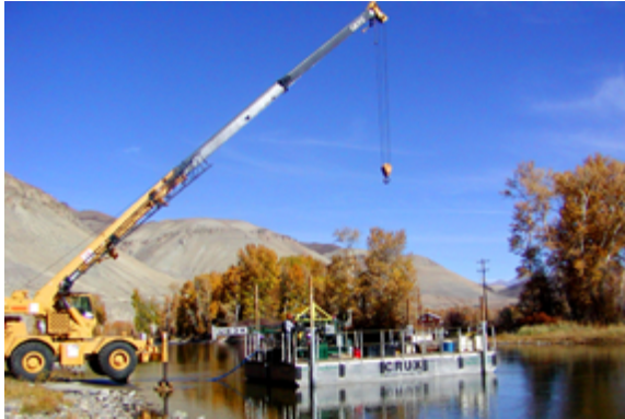
Performing geotechnical exploration work utilizing a Crux-owned specialty barge
