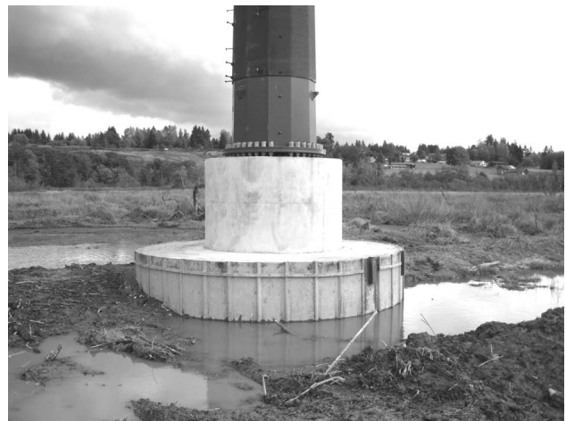
Figure 5 - Ebey Slough Micropile Deadend Foundation
