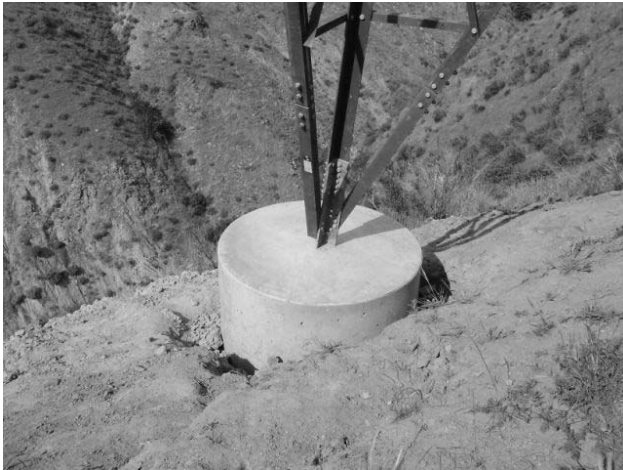
Figure 6 - TRTP Micropile Suspension Tower Leg Foundation
