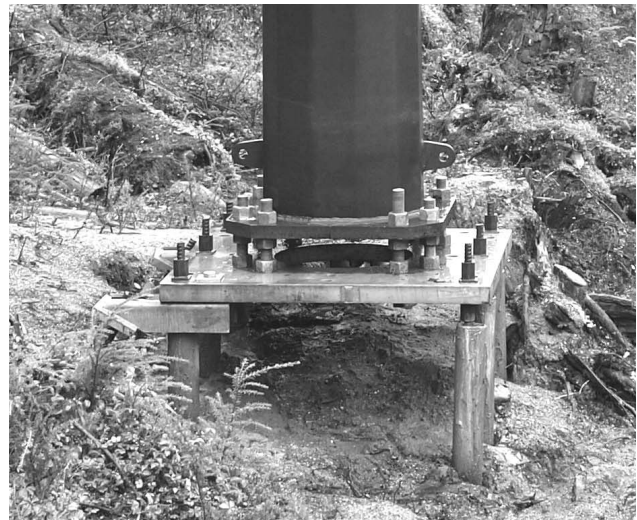
Figure 2 - Swan-Tyee Intertie Micropile Foundation
