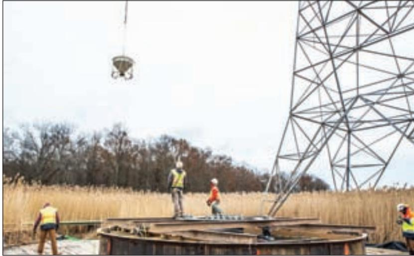
carriage were set on the cofferdam, and micropiles were installed in a battered array. Proof testing was then completed to confirm capacity. The micropile drill and drill carriage were removed from the site to allow for rebar installation and concrete form construction. A pre-constructed anchor bolt
