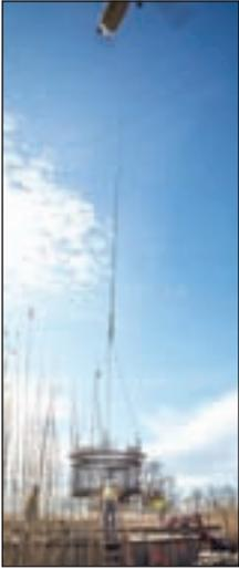
Left to right: ► closed-cell cofferdam set-up at each site. This set-up provided a stable platform for equipment in soft soils and groundwater, contained drill spoils from contaminating the wetland and acted as a form for concrete placement during pile cap construction. A speciality fabricated drill and rotating
