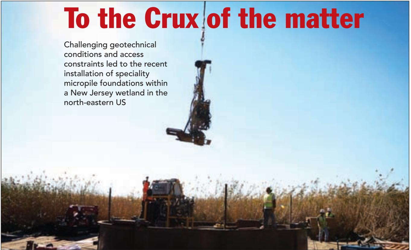
*Micropile drill delivered to site by helicopter*
