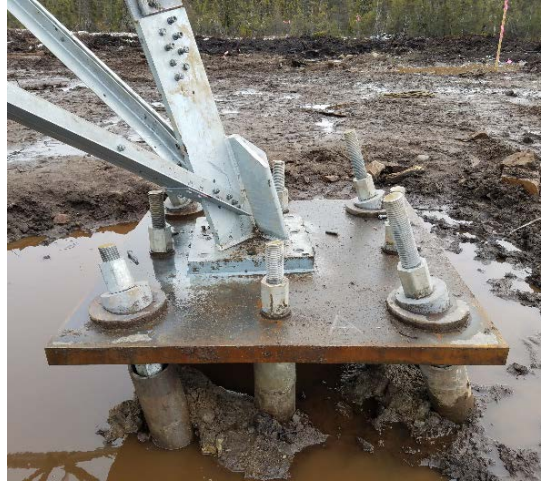
Figure 11. Installed D2/E1 steel cap micropile foundation
