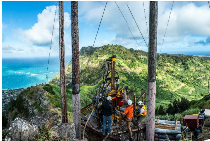
Figure 4. Micropile drill setup
