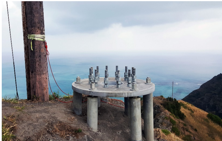
Figure 5. Completed steel cap micropile foundation
