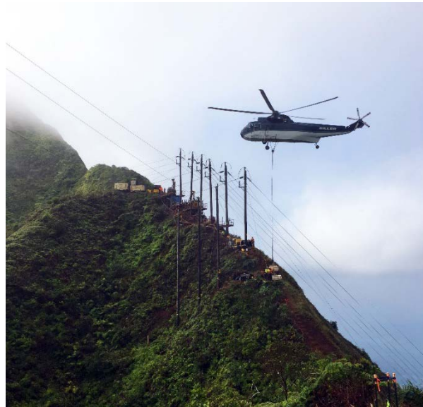
Figure 1. Replacement structures on steep ridgeline
