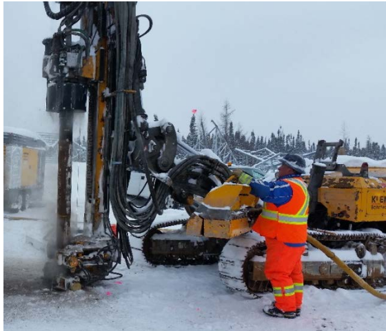
Figure 9. Micropile installation
