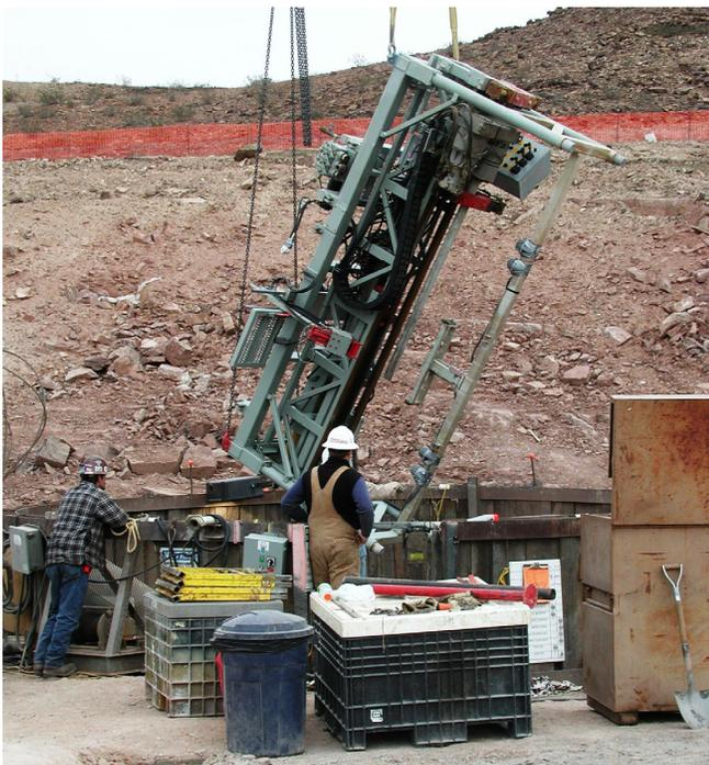
Figure 4. Lowering drill rig into Las Vegas Wash Tunnel north shaft
