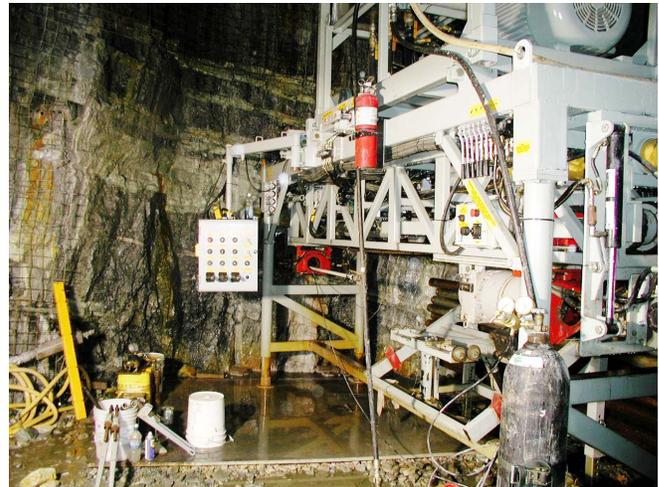
Figure 5. Horizontal drill rig set up in bottom of Las Vegas Wash Tunnel shaft
