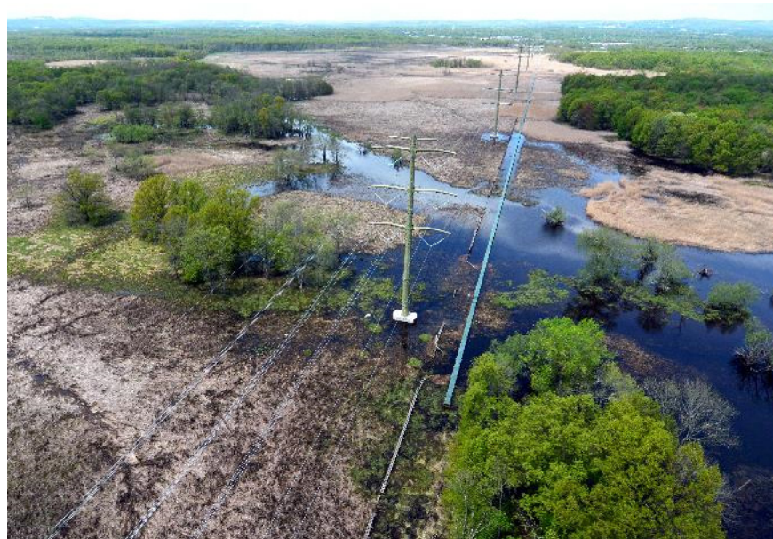
Figure 2: Completed Line Construction through Troy Meadows
