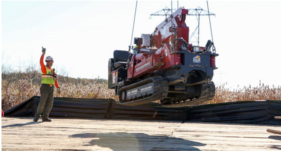
Figure 7: Helicopter Portable Crane Being Delivered to Site
