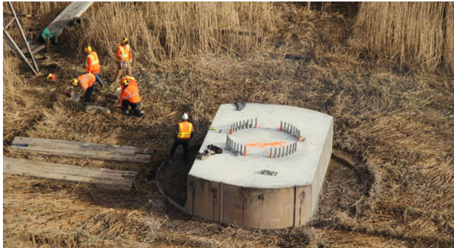
Figure 5: Value Engineered Concrete Pile Cap
