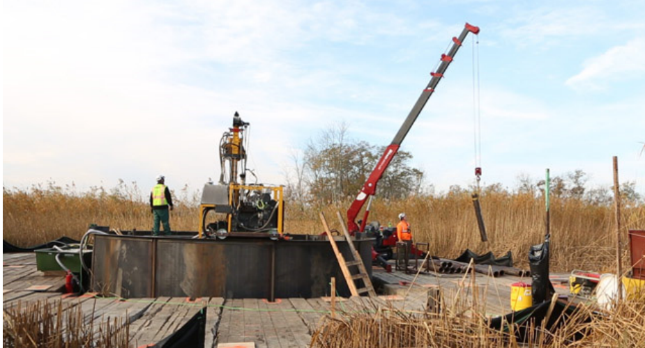
Figure 6: Drill Site Setup
