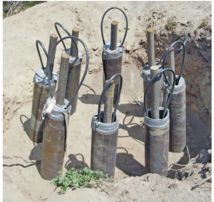
Micropiles being installed.
