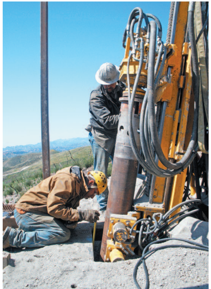
Micropiles being installed in a batter.
