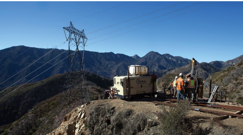
Micropile installation on the Tehachapi Renewable Transmission Project (patent-pending spin drill)
