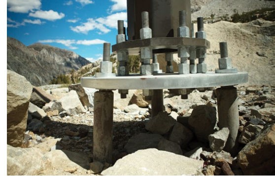
Completed steel cap micropile foundation on the Rhinedollar Distribution Project
