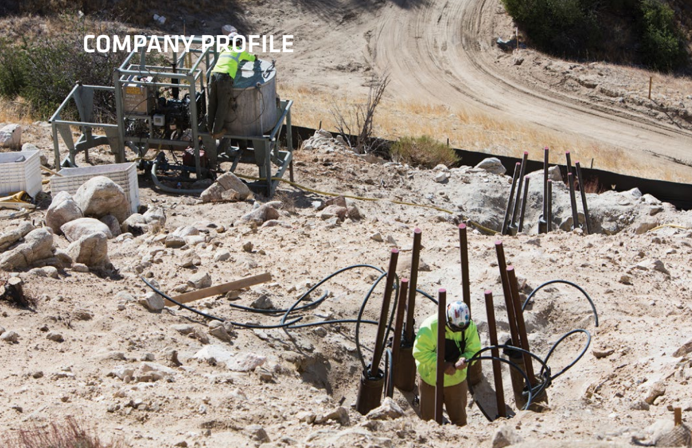
Micropile foundations are grouted on the Tehachapi Renewable Transmission Project
