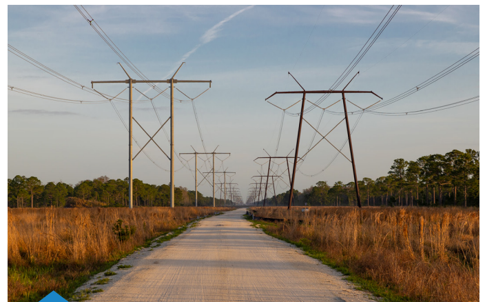
OLD VS NEW FPL 500KV STRUCTURES
