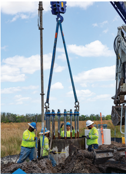
ALIGNING THE ANCHOR BOLTS
