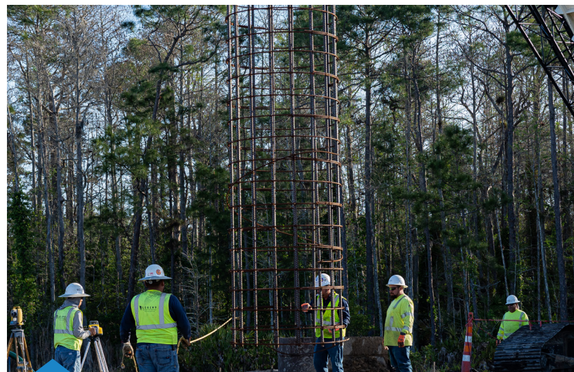
LIFTING THE CAGE
