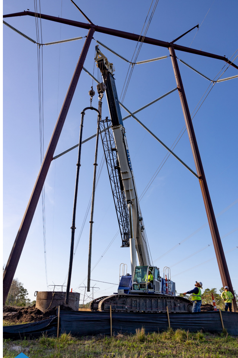
PUMPING CONCRETE INTO THE HOLE
