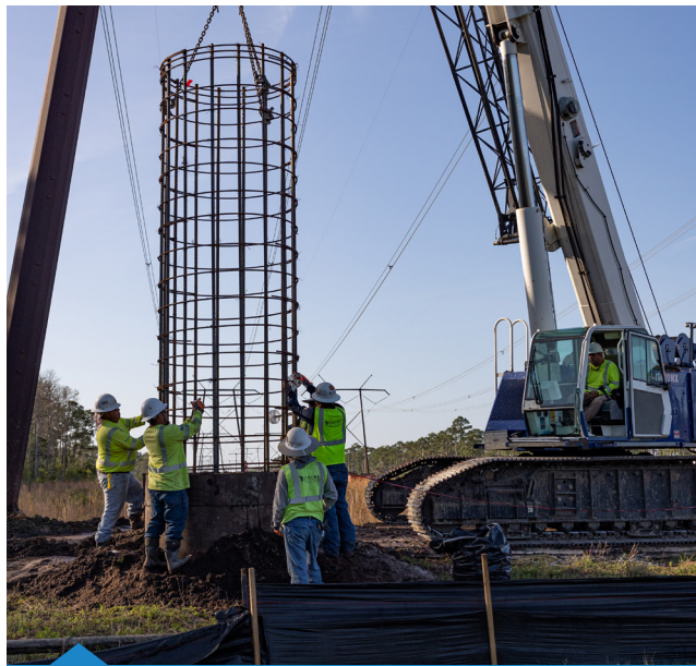
LIFTING THE CAGE
