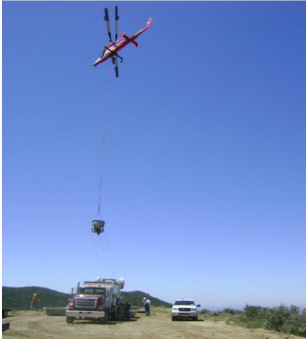
Figure 12: A K-Max helicopter transports volumetric concrete to the tower site.
