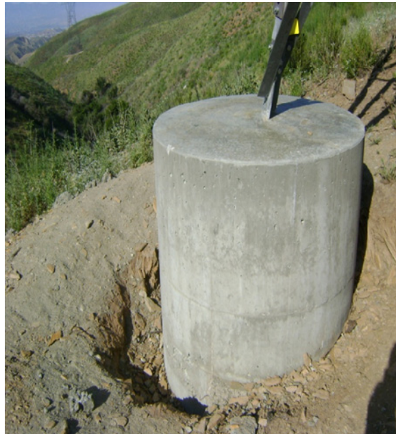
Figure 5: A complete micropile foundation is indistinguishable from other types on the surface.
