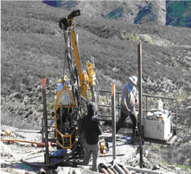
Figure 9: Micropile drill platform and drill rig.
