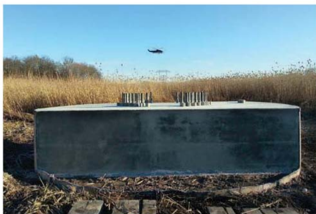
Completed micropile foundation prior to setting monopole.
