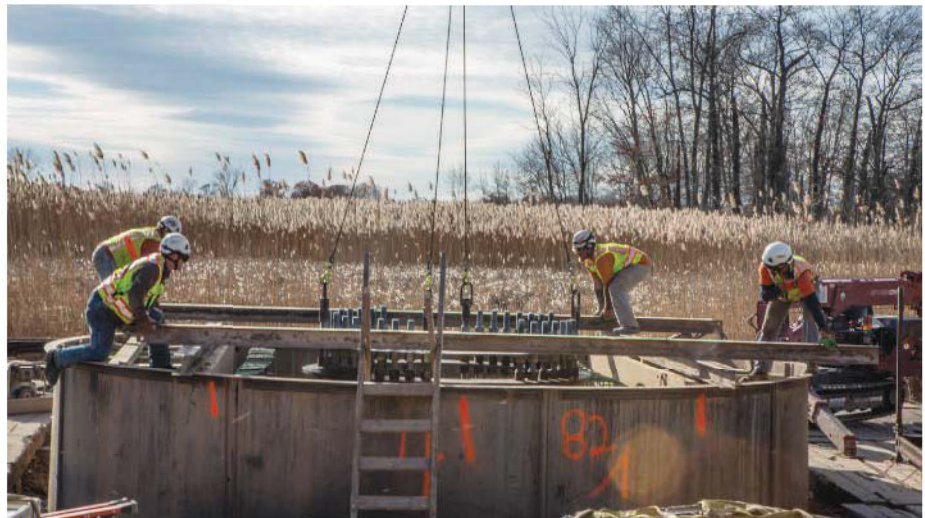
This crew is working on the precise setting of the anchor-bolt cage.
