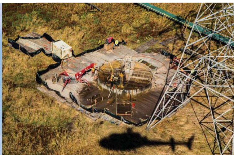
Cofferdam setup contained drill spoils from entering the wetland.
