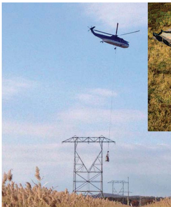
Micropile drills were transported to structure locations by helicopter.
