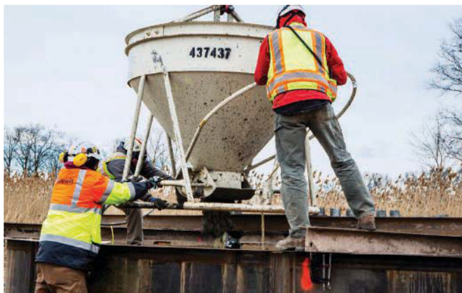
Helicopter-assisted concrete pouring for micropile caps.
