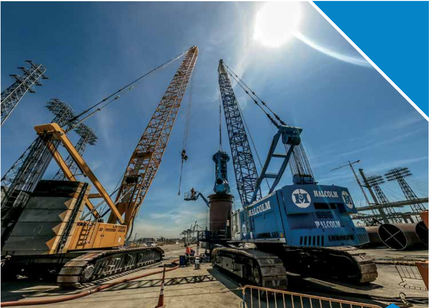
SPHERICAL GRAB EXCAVATION
