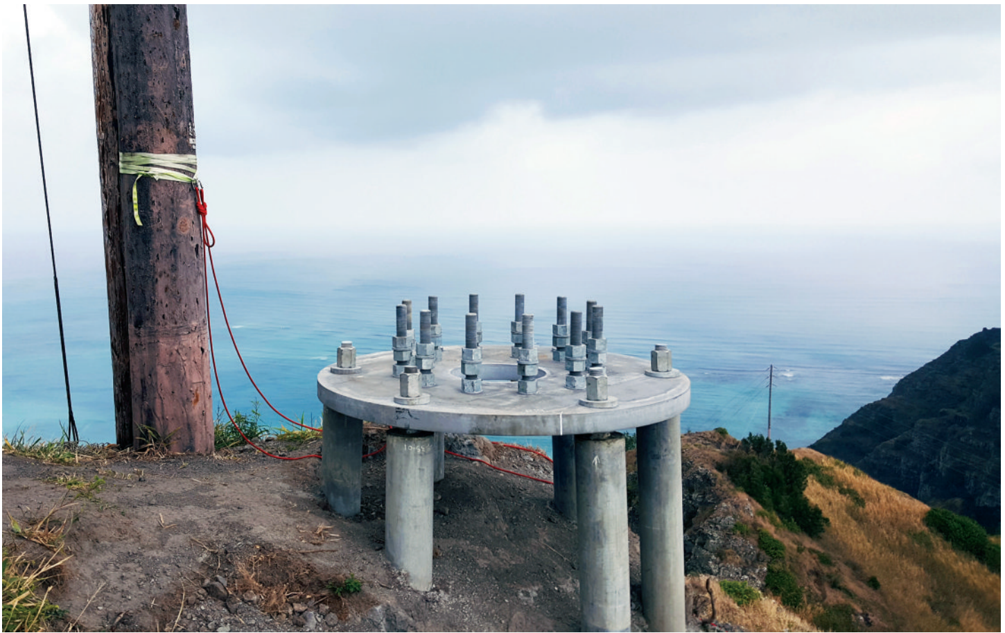
Completed steel cap micropile foundation
