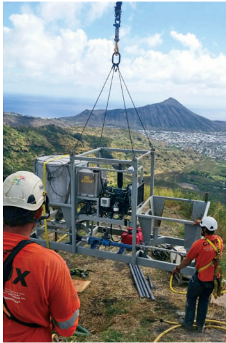
Grout plant being delivered to the site by helicopter
