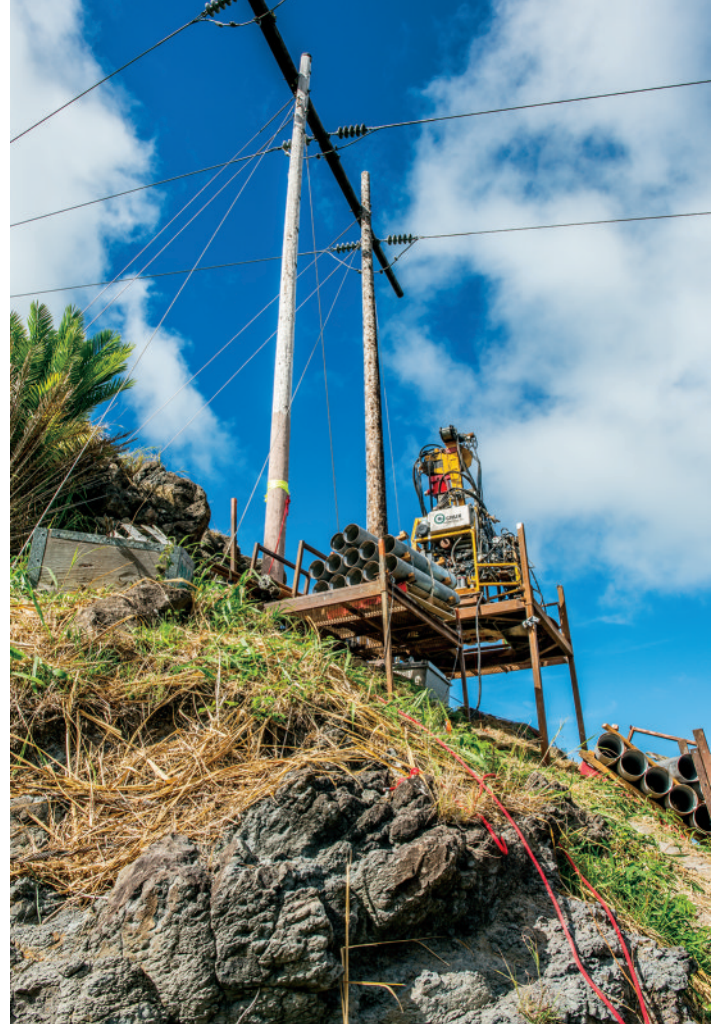
Drilling micropiles underneath in-service lines
