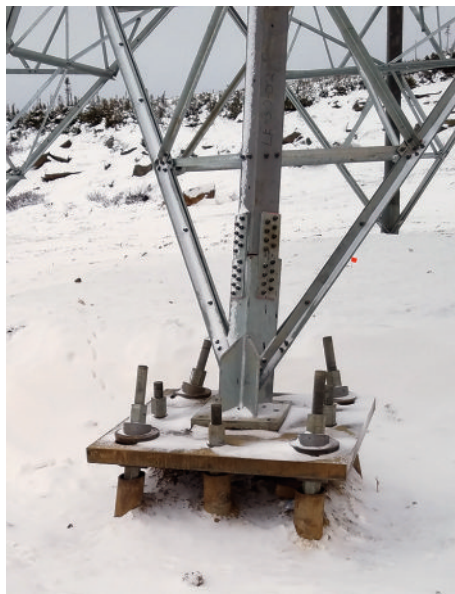
Steel pile caps installed in snow
