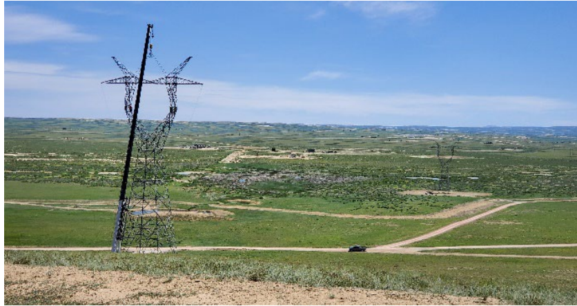
Figure 6. Tower Erection on Completed Foundation
